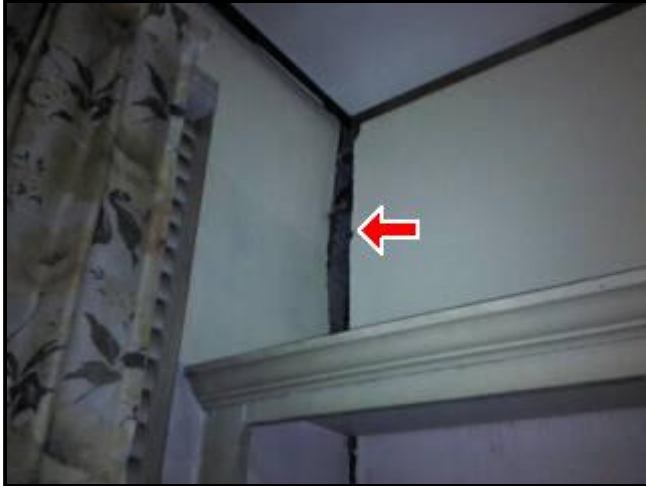
4.1 Picture 1 first floor north
