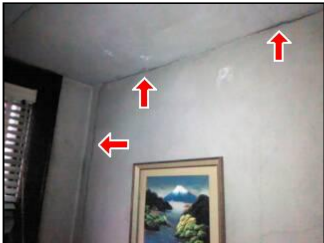
4.1 Picture 3 third floor walls and ceiling
