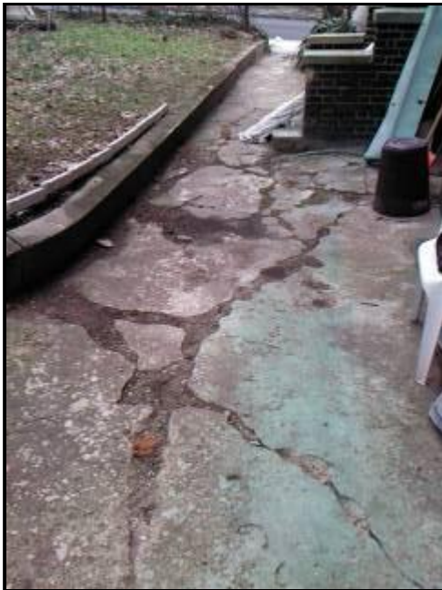
2.4 Picture 1 rear walkway concrete
