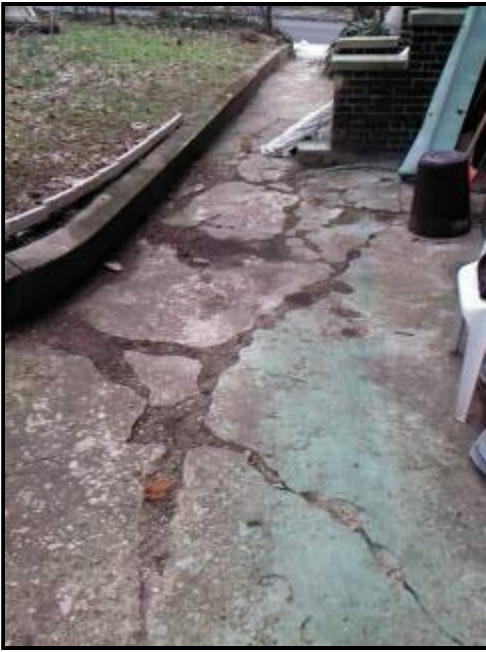
2.4 Picture 1 rear walkway concrete
