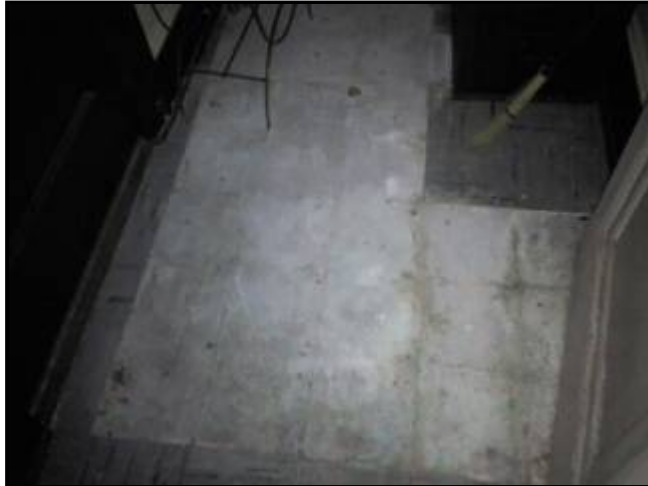
4.2 Picture 2 floor behind kitchen
