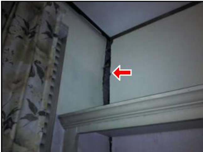
4.1 Picture 1 first floor north
