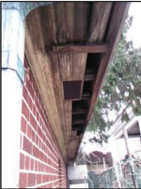
2.6 Picture 1 garage eave
