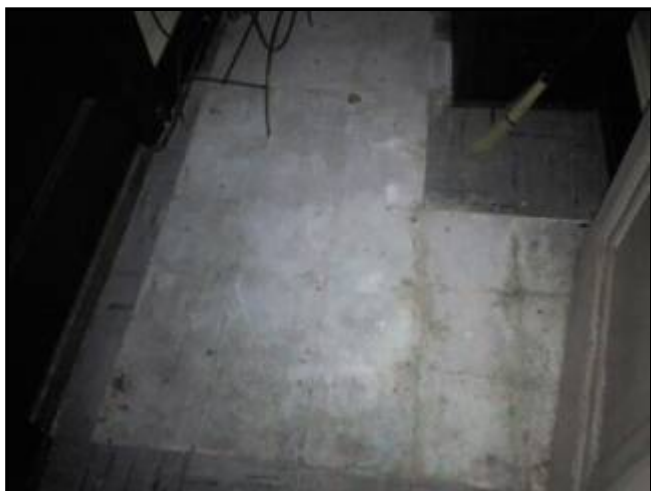
4.2 Picture 2 floor behind kitchen
