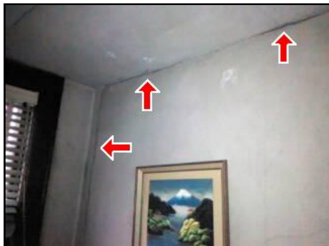
4.1 Picture 3 third floor walls and ceiling
