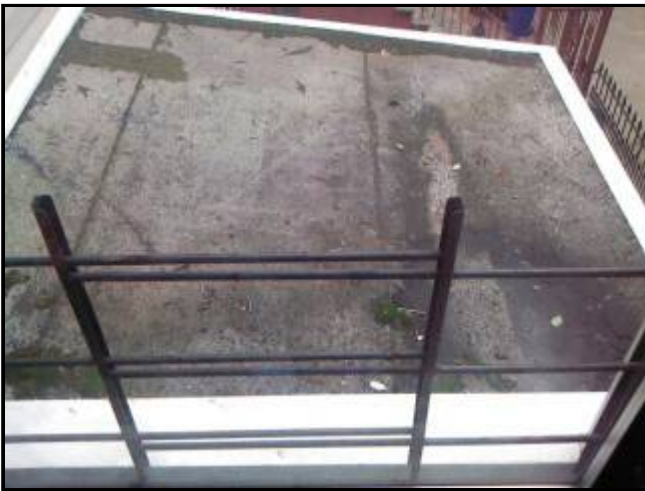
1.0 Picture 1 front roof
