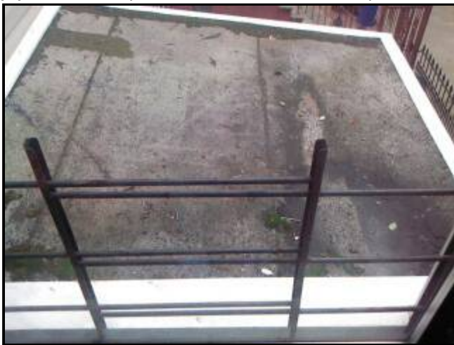
1.0 Picture 1 front roof
