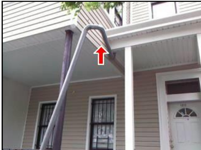
1.3 Picture 1 roof drain
