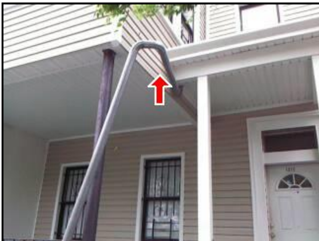
1.3 Picture 1 roof drain
