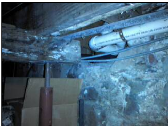
4.2 Picture 1 main beam cut to allow drain
