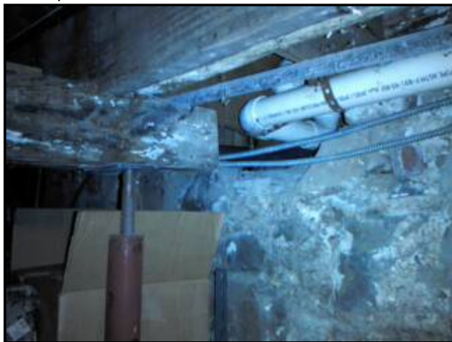
4.2 Picture 1 main beam cut to allow drain
